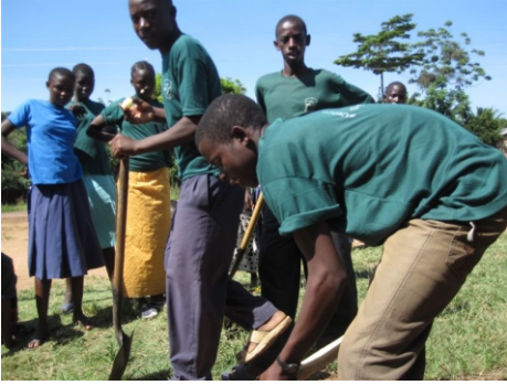
DIGGING 2 KM TRENCH WITH HELP FROM PUPILS AND EVEN PRISONERS
