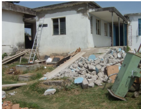
AN ABANDONED BUILDING WAS PLACED AT OUR DISPOSAL.
